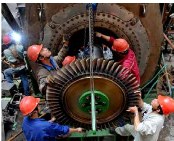
FIGURE 4. Energy Conservation Retrofit in a Power Plant
