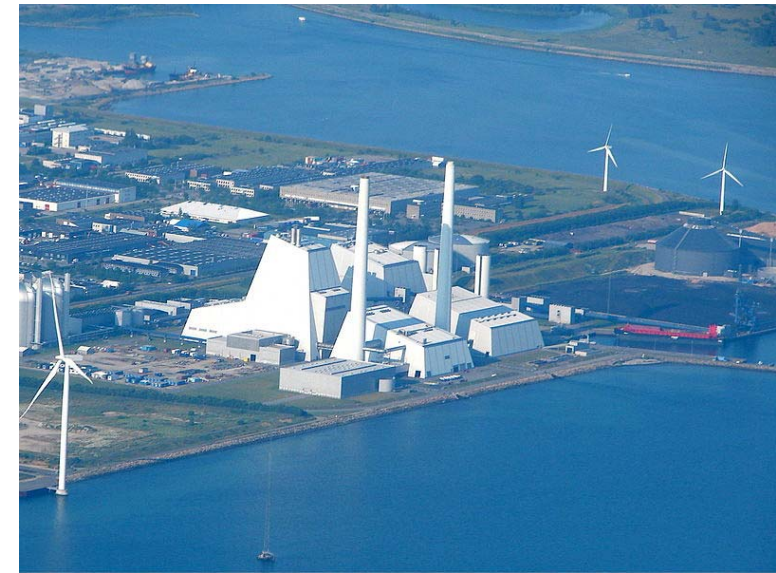
Avedøreværket, a combined heat and power plant
